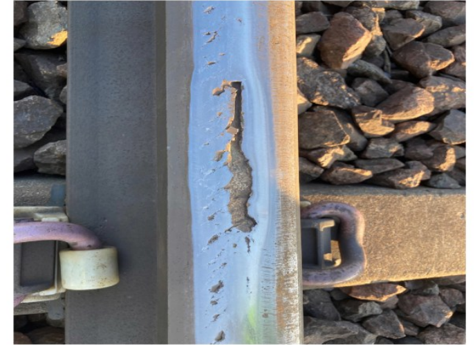
Low rail RCF damage on a curve (H-Nia et al, 2023)
